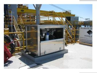
Each MARS Offshore 316L SS Cabinet Enclosure features removable panels, half-panel drop doors, seal-welded containment pans & provisions for locking. Optional 316L SS roller shutter doors available upon request.
